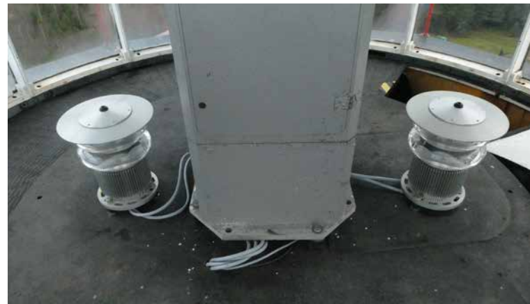
Sabik E8278 standby lanterns, photograph by T. Rosenberg.
