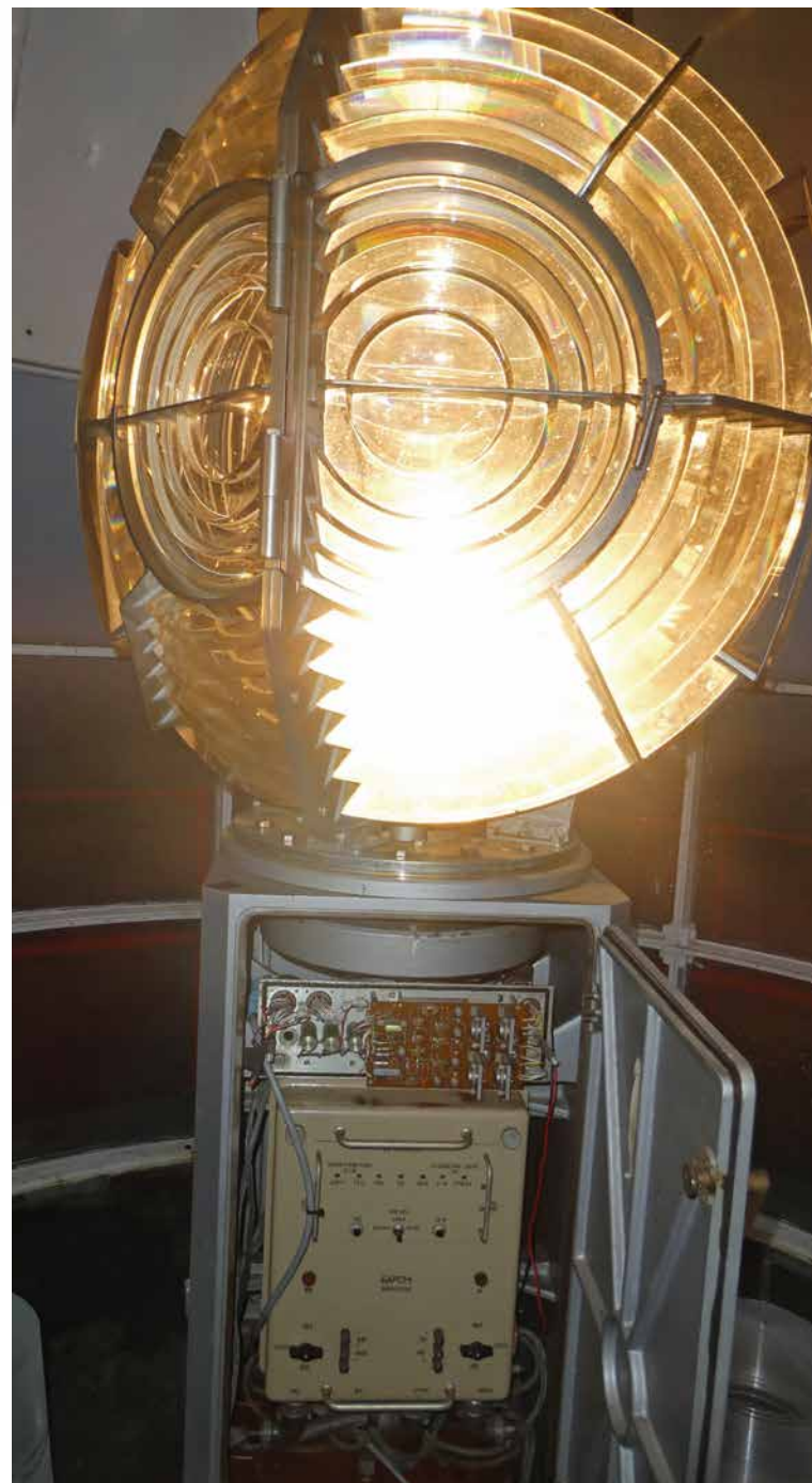
The powerful Soviet-manufactured EMV-930 lighting apparatus with a rotating Fresnel lens, in operation from 1981 to 2020, photograph by T. Rosenberg.
