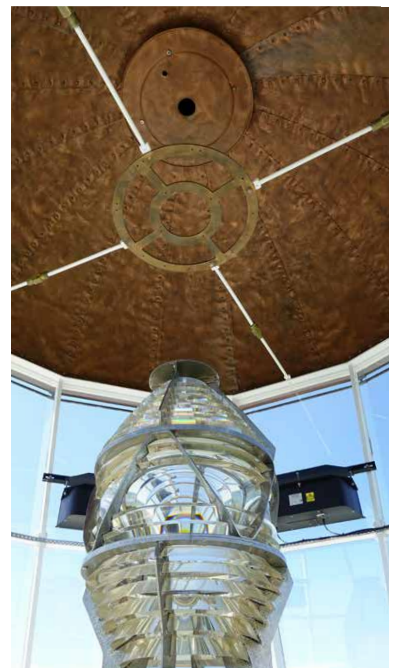
On the foreground: the Chance Brothers & Co lighting device installed in 1870. In the background: the modern Sabik light system lanterns. Photo from the year 2021, T. Vilu
