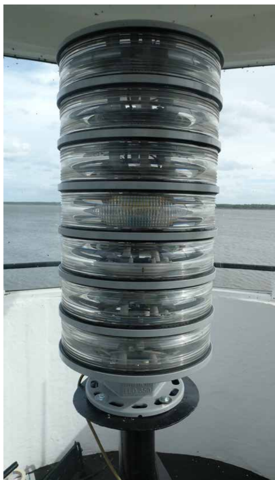
The first lighthouse's first LED light: Sabik LED-350-7W omnidirectional lantern in the Mehikoorma lighthouse, photo T. Vilu
