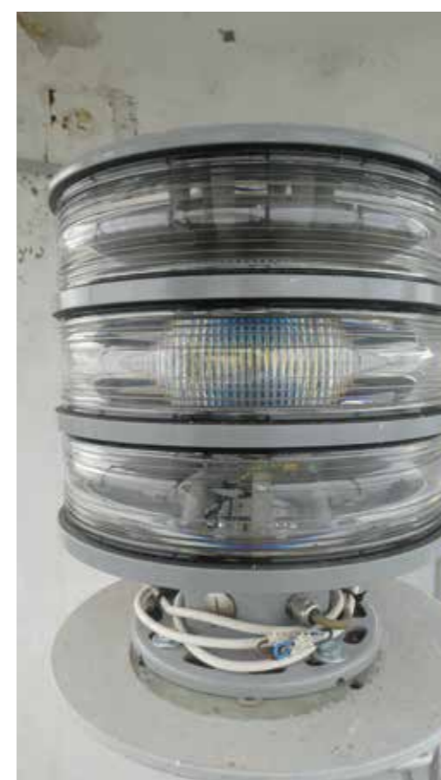
The first LED lantern (Sabik LED350-4) in Nina Lighthouse, photo T. Vilu
