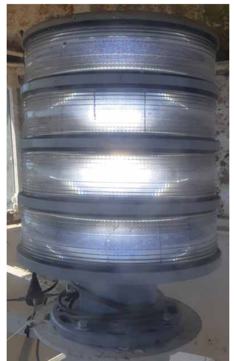
Rannapungerja Lighthouse's first LED lantern (Sabik LED350-4), photo T. Vilu
